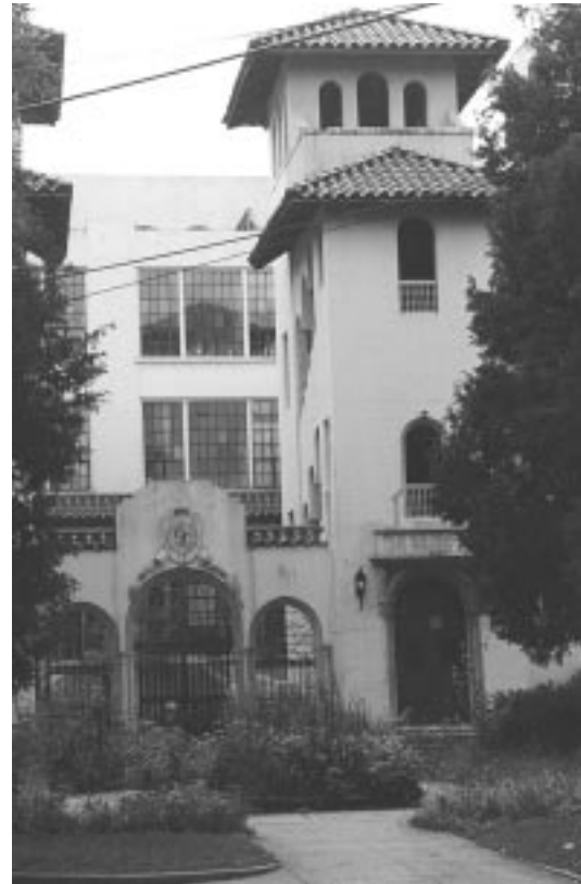
This former cigar factory in Trenton was converted into apartments.
