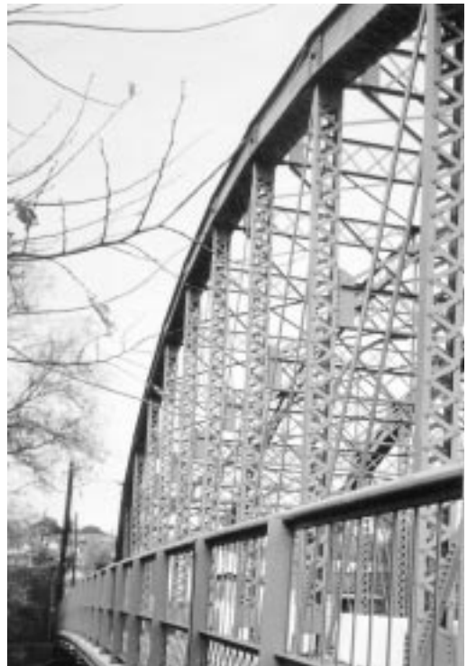
The Arch Street bridge over the Passaic River in Paterson was built in 1905 and restored in 1997.
