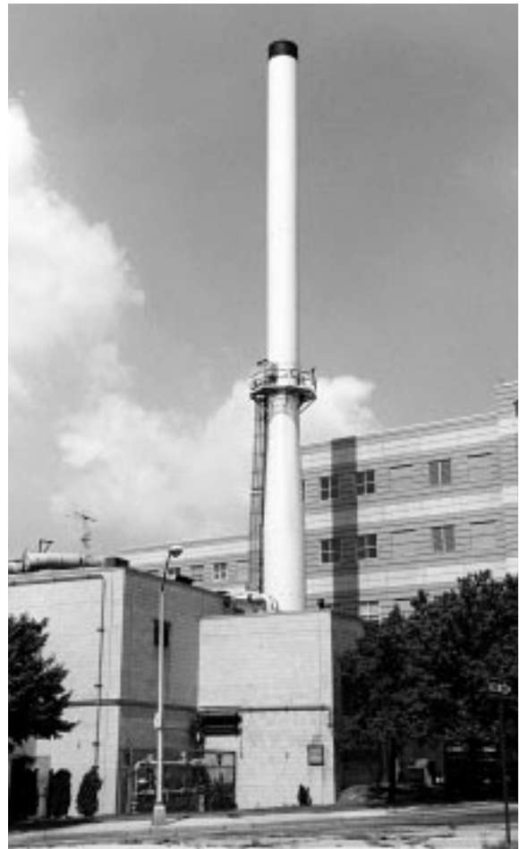
A cogeneration plant in Trenton.
