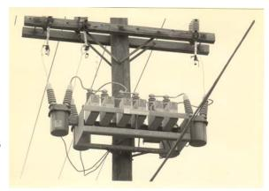
**Figure 4-3.** Six large high voltage capacitors.
