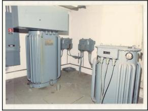
Figure 4-1. Two PCB Transformers.
