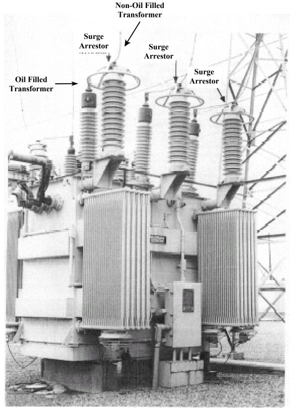
Figure 4-2. Oil filled and non-oil filled transformers.
