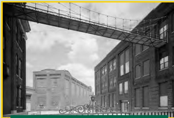
The view of NJHMFA's building from S. Broad Street as the building appeared before renovation.
