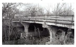
Route 27 (Lake Avenue) Bridge over LVRR, Metuchen, New Jersey in 2007 (Source: RGA files). This concrete-encased steel stringer bridge was the preferred bridge type of the State Highway Department between the two world wars.
