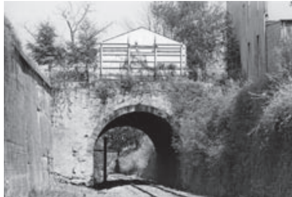
Railroad Underpass, Farnsworth Avenue, Bordentown, Burlington County
