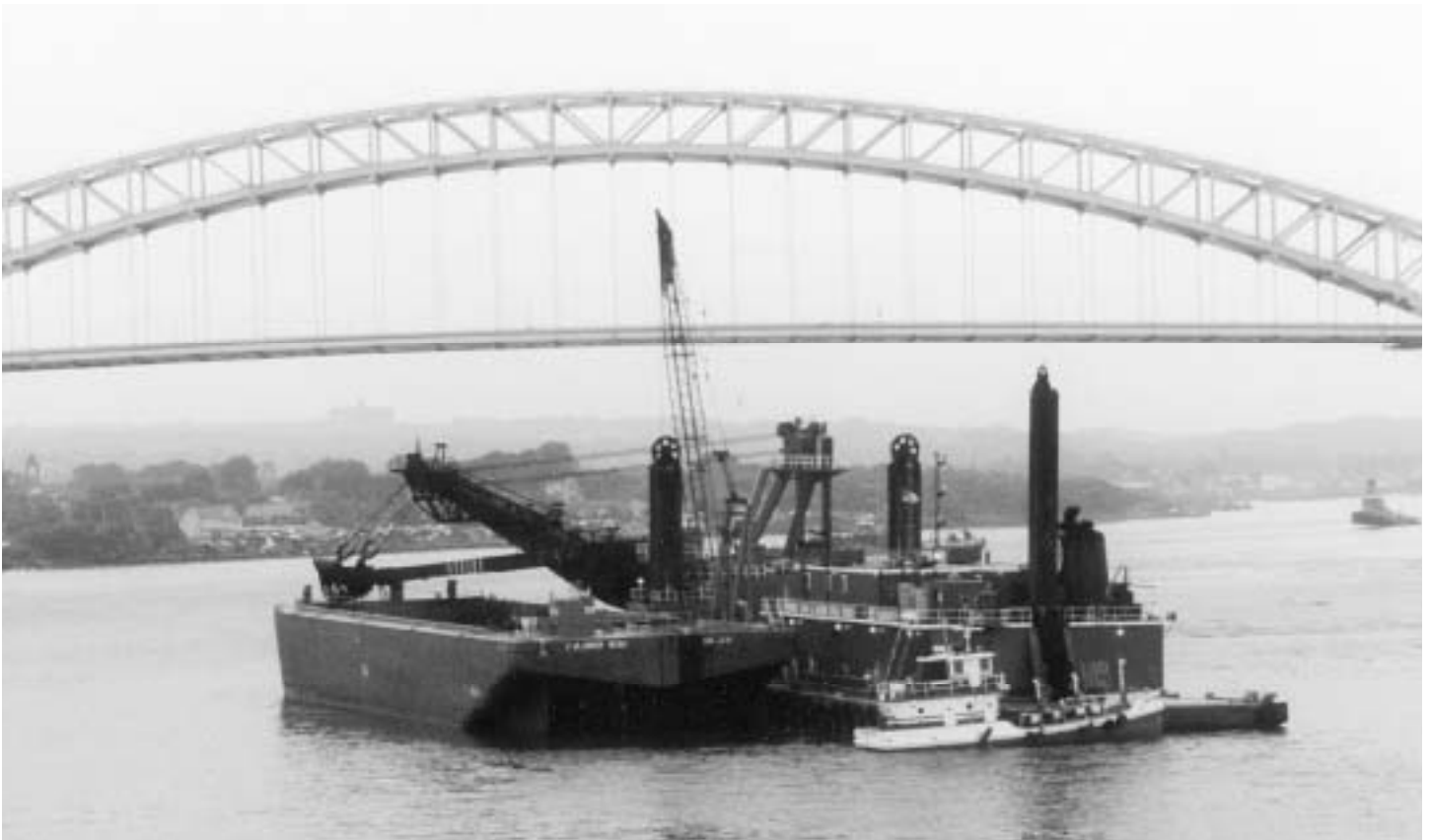
A massive dredge loads a scow with bedrock blasted from the Kill Van Kull.
