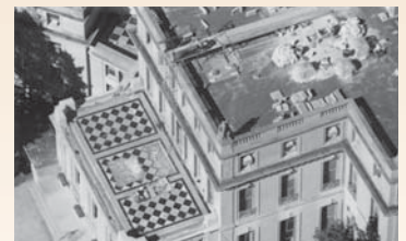
In progress: Roof Restoration
