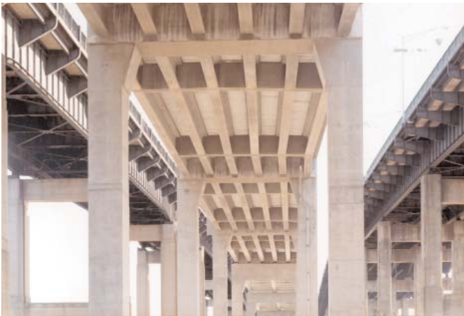
Garden State Parkway and Route 9 Bridges after Widening of Route 9 Note lower profile (top), pier changes (middle), and framing (bottom).
