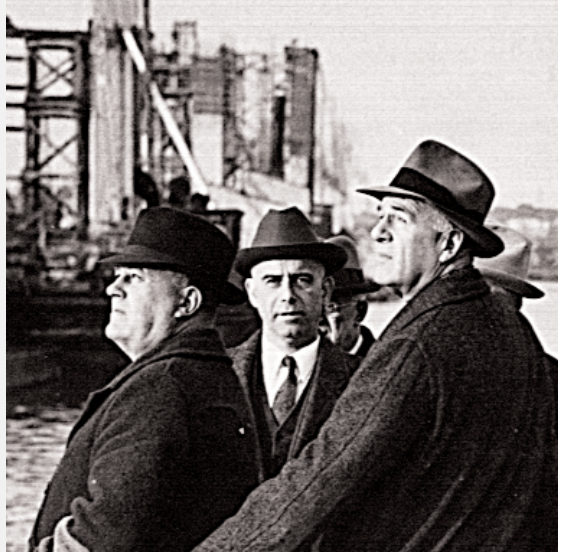
Morris Goodkind (facing camera) inspecting construction of Edison Bridge, 1939.
