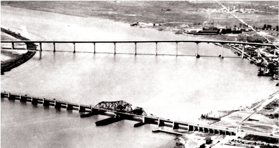
Victory Bridge, in foreground, is a swing bridge, pivoting on a center pier to allow boat traffic to pass through two channels. Opening the bridge in the summer resulted in huge traffic backups. Edison Bridge, west of the Victory, was built high enough to allow all vessels to pass under. Source: NJDOT
